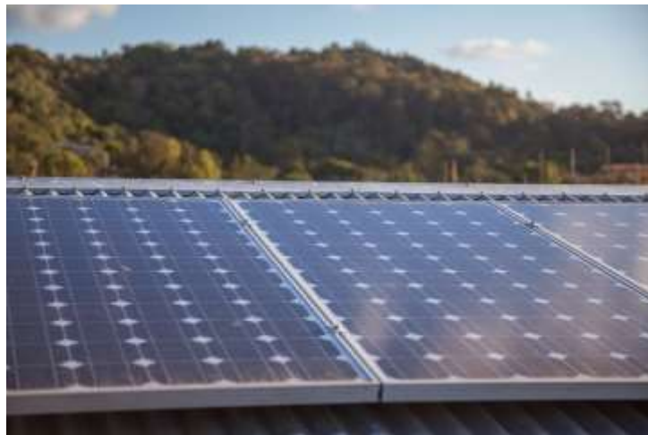
The shift to more sustainable energy sources means developing appropriate controls to maintain reliability. Image: Sander Van Dijk
